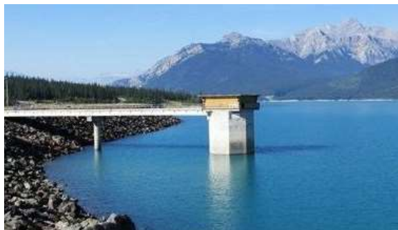
Figure 15. Bighorn Dam intake head gate house
