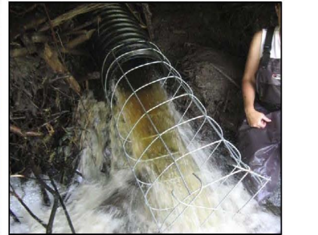
6. Protecting the end
