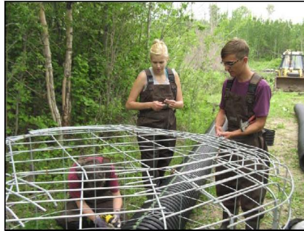
2. Attaching pipe to cage
