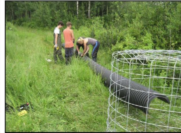
3. Joining the pipes
