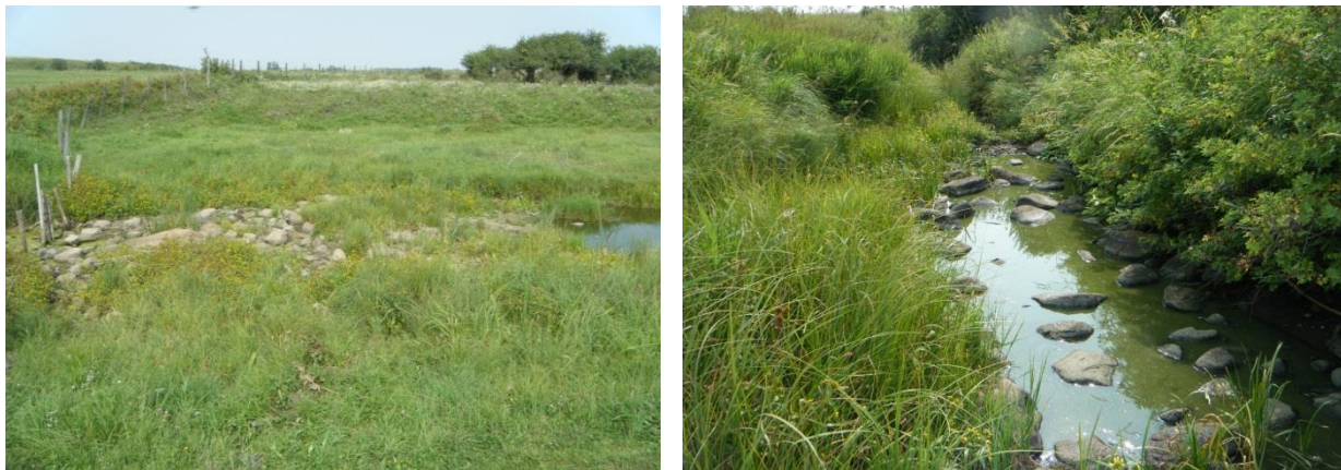
Figure 29: A ford (left) blocking stream channel (right) (CPPENV 2015).
