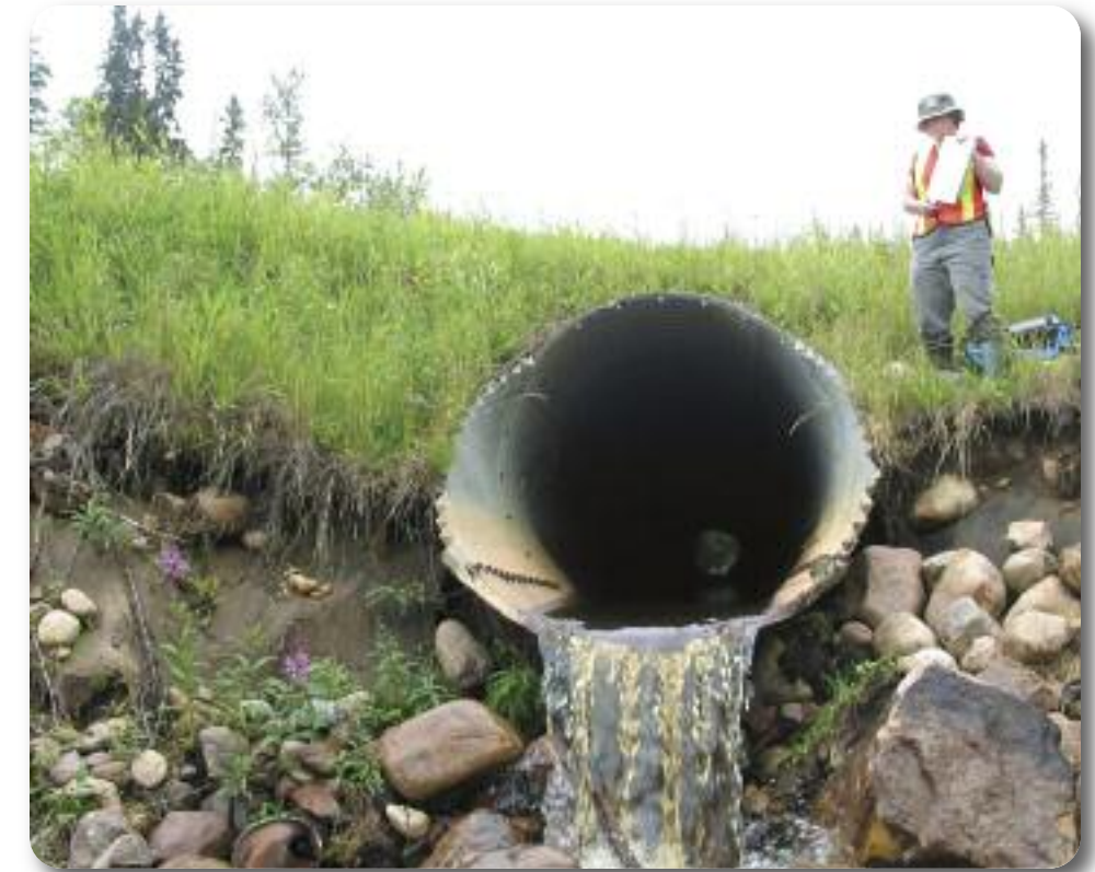
An example of a hanging culvert.
