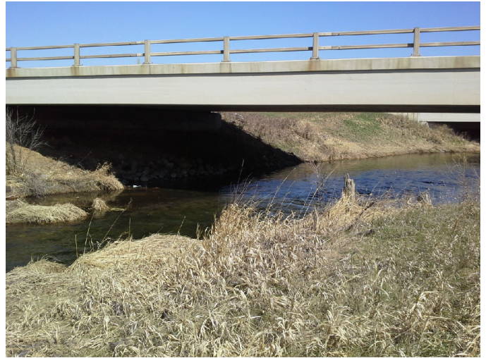
Photo No.: Photos-20180511-183939.jpg Description: Inlet
