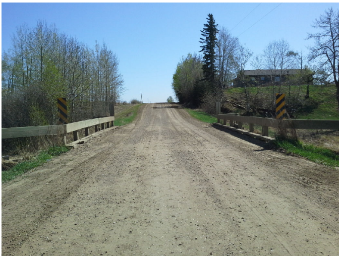
Photo No.: Photos-20180511-181206.jpg Description: Deck
