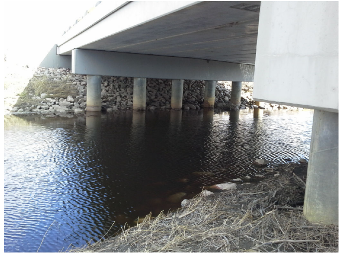
Photo No.: Photos-20180508-213901.jpg Description: Inlet
