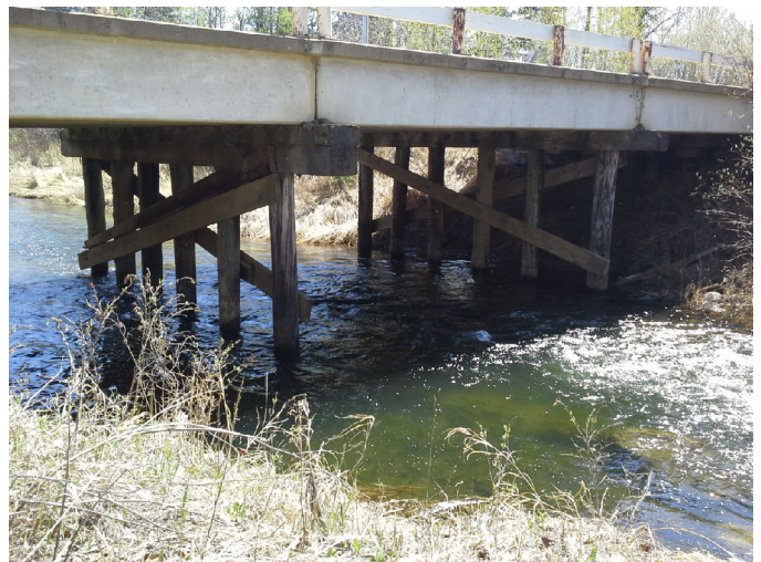
Photo No.: Photos-20180511-191311.jpg Description: Inlet
