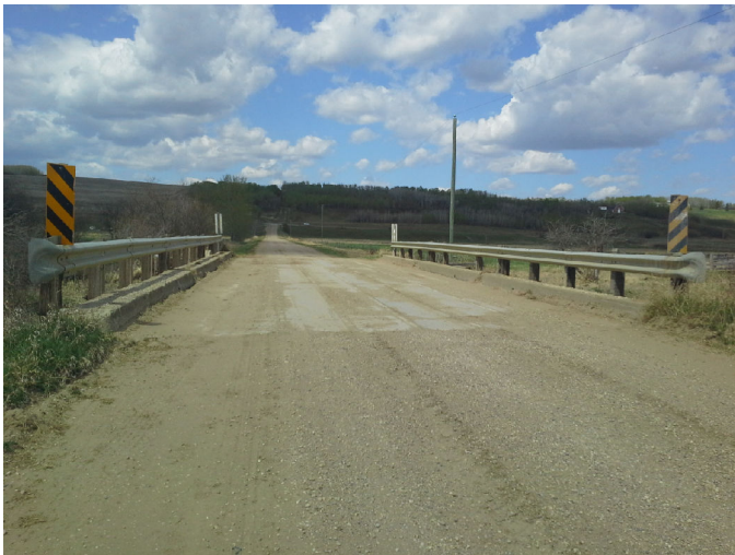
Photo No.: Photos-20180511-211314.jpg Description: Deck
