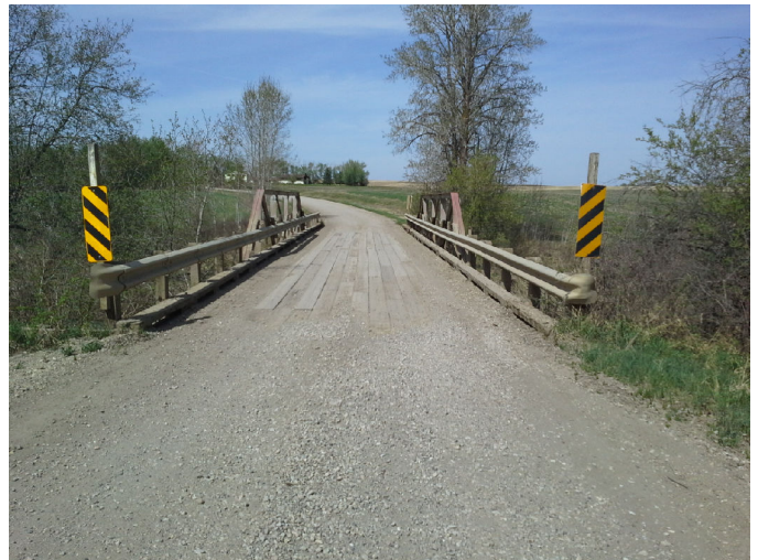
Photo No.: Photos-20180514-212529.jpg Description: Deck
