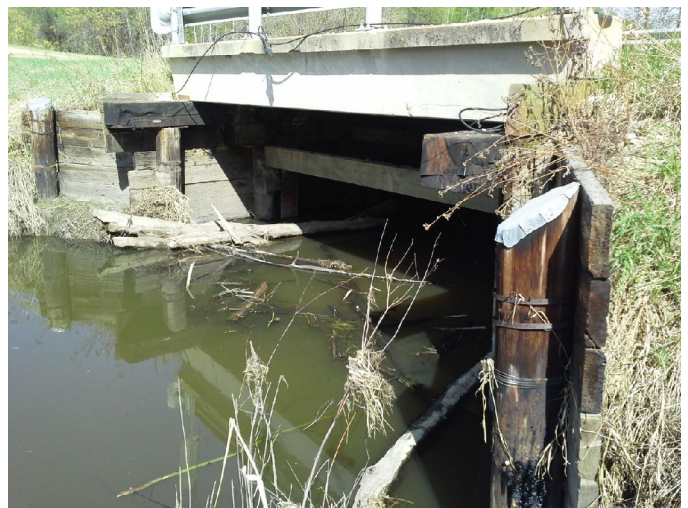
Photo No.: Photos-20180514-171424.jpg Description: Inlet
