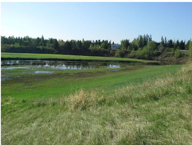
Photo No.: Photos-20180518-145855.jpg Description: Downstream
