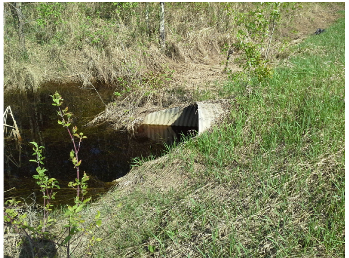
Photo No.: Photos-20180518-165807.jpg Description: Culvert 1 - Outlet
