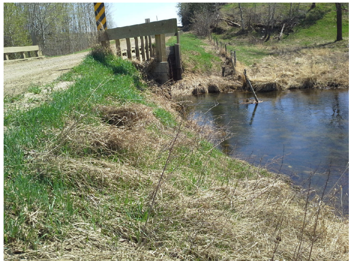
Photo No.: Photos-20180511-181239.jpg Description: Possible erosion from road to bank
