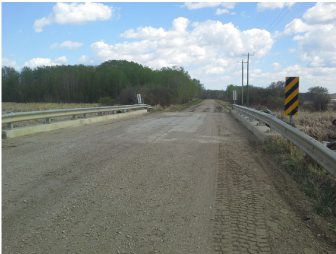
Photo No.: Photos-20180511-212849.jpg Description: Deck
