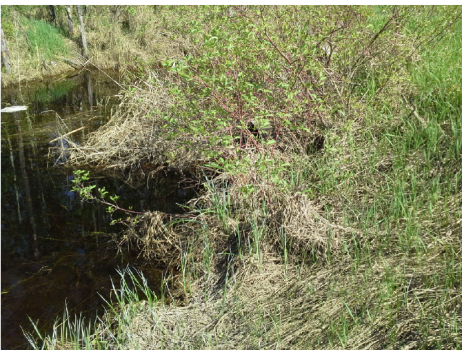
Photo No.: Photos-20180518-165830.jpg Description: Culvert 2 - Outlet
