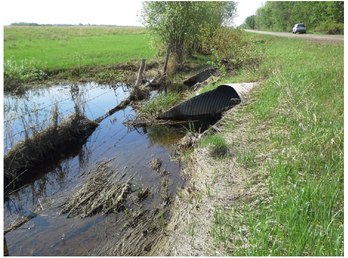
Photo No.: Photos-20180518-165658.jpg Description: Inlet
