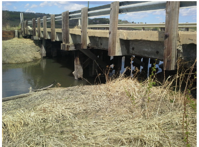
Photo No.: Photos-20180511-211351.jpg Description: Inlet
