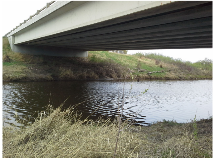
Photo No.: Photos-20180516-200102.jpg Description: Inlet
