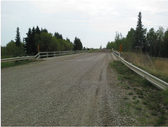
Photo No.: Photos-20180516-204223.jpg Description: Deck
