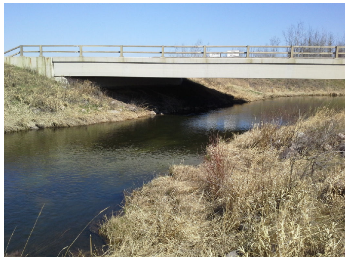
Photo No.: Photos-20180511-184145.jpg Description: Downstream
