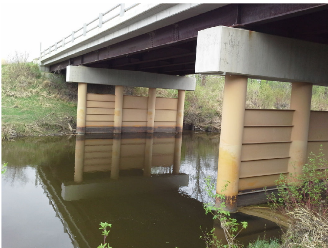
Photo No.: Photos-20180516-204542.jpg Description: Inlet
