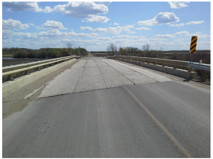
Photo No.: Photos-20180508-212500.jpg Description: Deck
