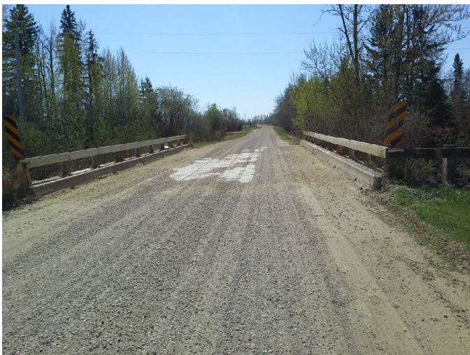
Photo No.: Photos-20180511-191249.jpg Description: Deck
