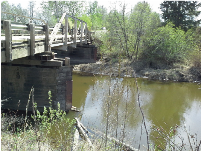
Photo No.: Photos-20180514-212410.jpg Description: Inlet
