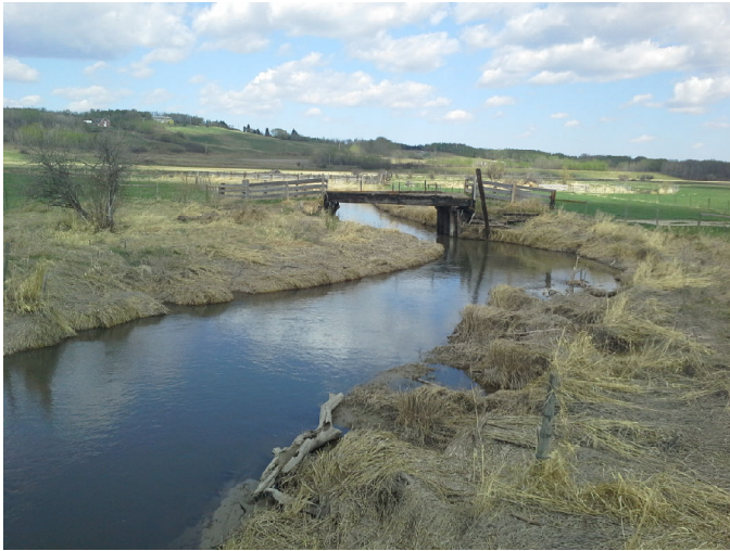
Photo No.: Photos-20180511-211227.jpg Description: Downstream
