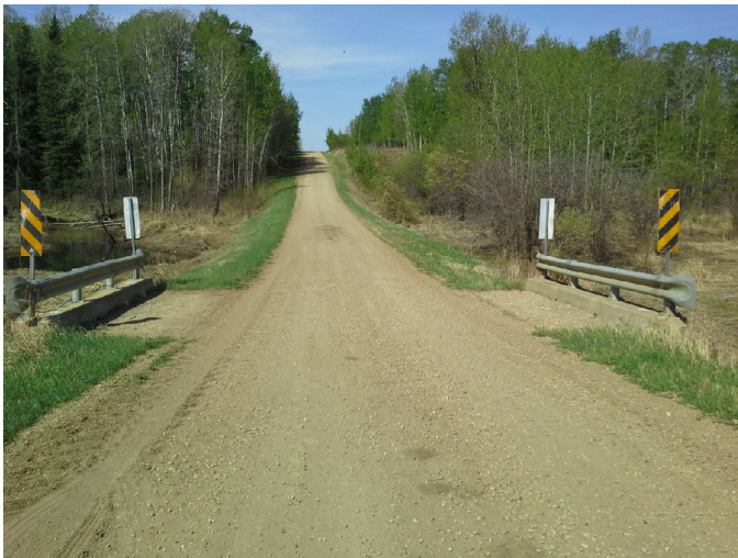
Photo No.: Photos-20180514-171213.jpg Description: Deck
