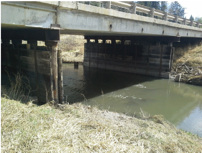
Photo No.: Photos-20180511-204529.jpg Description: Inlet
