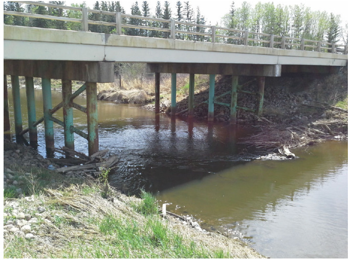
Photo No.: Photos-20180514-213844.jpg Description: Inlet
