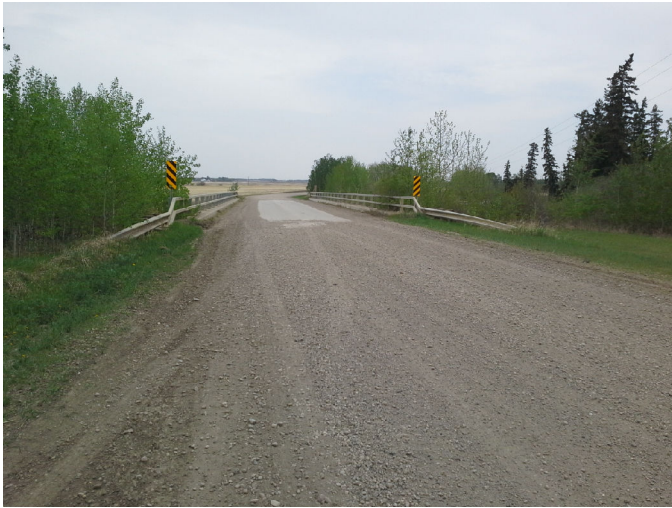
Photo No.: Photos-20180516-202230.jpg Description: Deck
