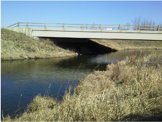
Photo No.: Photos-20180511-184919.jpg Description: Inlet
