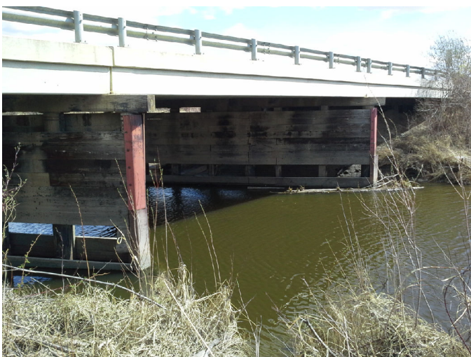
Photo No.: Photos-20180508-212638.jpg Description: Inlet
