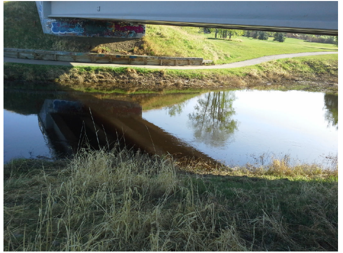
Photo No.: Photos-20180518-145736.jpg Description: Inlet
