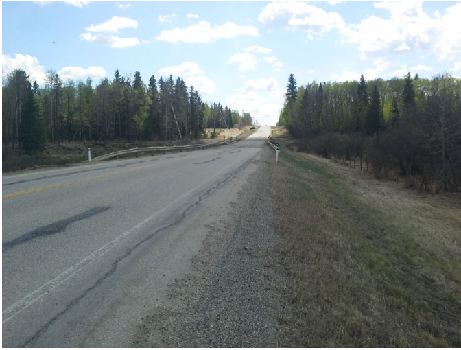
Photo No.: Photos-20180511-204314.jpg Description: Deck
