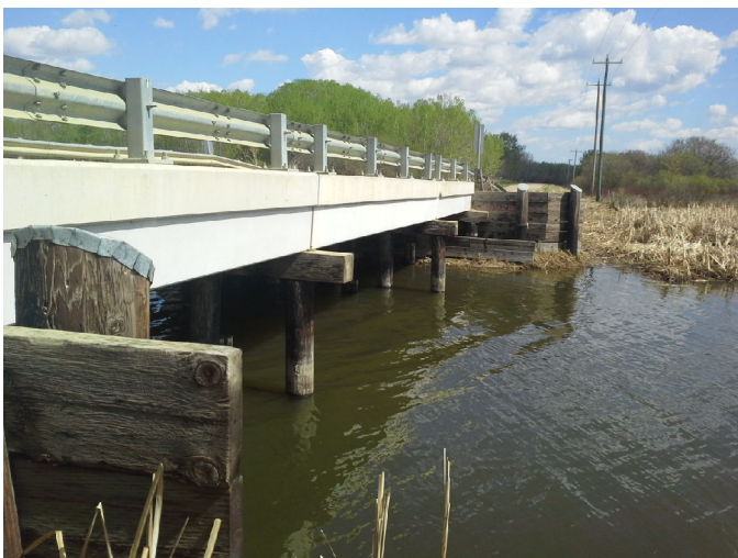
Photo No.: Photos-20180511-212930.jpg Description: Inlet
