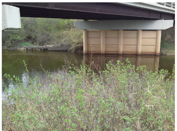
Photo No.: Photos-20180516-202731.jpg Description: Inlet
